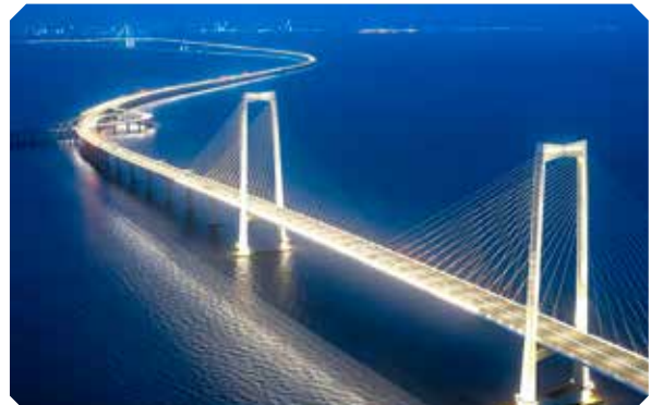
▶ Shenzhen-Zhongshan Corridor Lighting Project
