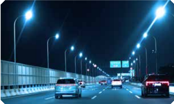
▶ Shanghai Urban Road Lighting Project
