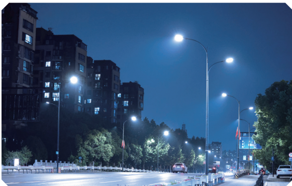
► Hangzhou Urban Road Lighting Project
