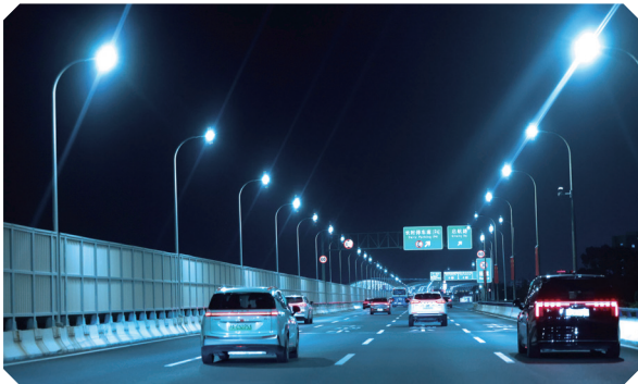
► Shanghai Urban Road Lighting Project
