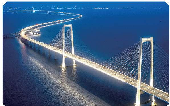
► Shenzhen-Zhongshan Corridor Lighting Project
